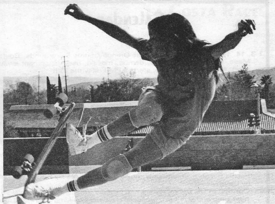
Station to station air born connection via Skitch Hitchcock's ramp. Photo by Ruiz.
